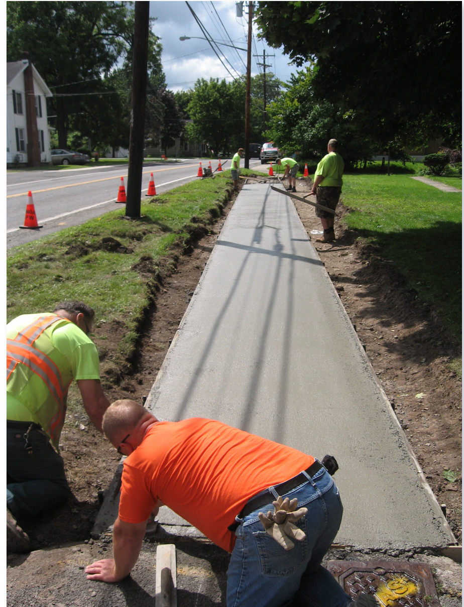
Inserting sidewalks on Main Street
